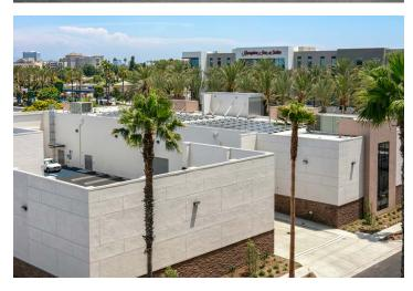
Due to the substation's proximity to Disneyland Resort, special provisions were required for the final design to control noise and hide all substation equipment from street and rooftop view. All incoming/outgoing electric lines to the substation were constructed underground to ensure the building remained aesthetically pleasing.
